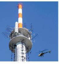
ried out by a conventional helicopter, as you have to measure very close to the antenna. The radiation aperture is also very close to the near horizon and the sites are normally established in populated areas.
